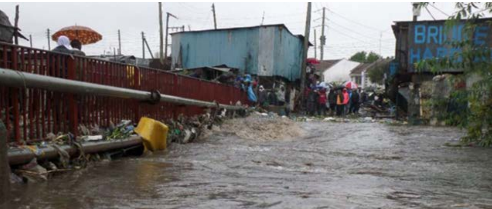
Figure 16 Hazina/Kaiyaba bridge flood Source: Daily Nation
