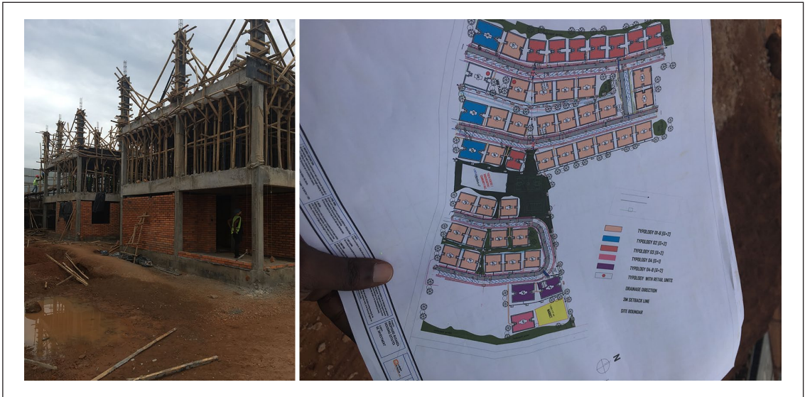
PHOTO 2A AND 2B Construction on the resettlement site of Busanza
