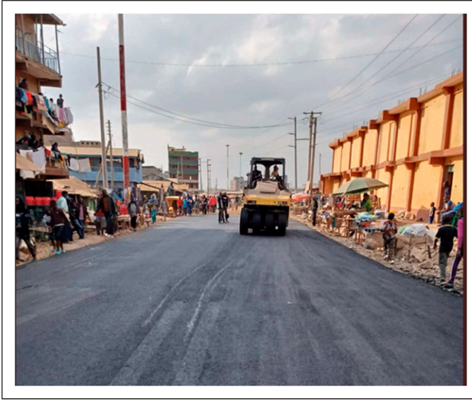
Figure 5. A new improved Road in Mukuru. Credit: J. Corburn.
