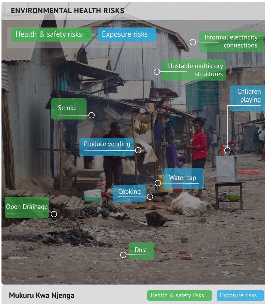
FIGURE 3. EXISTING CONDITIONS: ENVIRONMENTAL & HEALTH RISKS IN MUKURU
